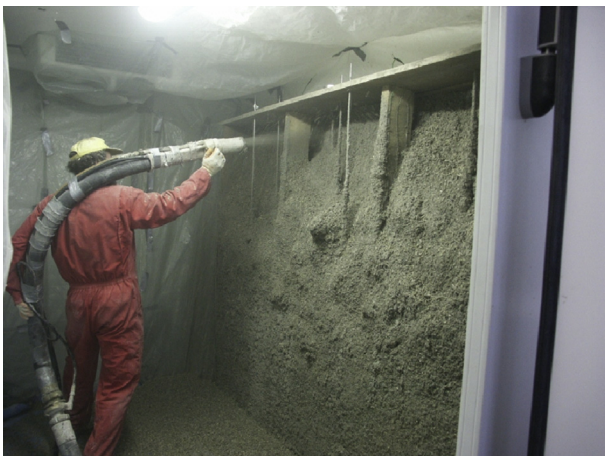
Fig. 1. Projected hemp concrete.
