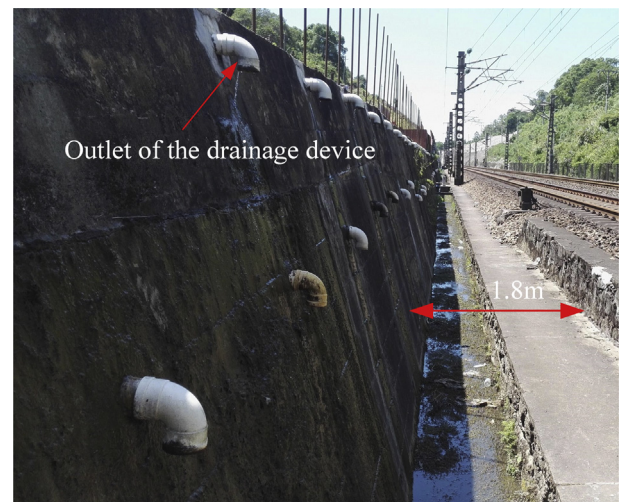
Fig. 2. Implementation of the drainage device at Beijing-Guangzhou railway.
