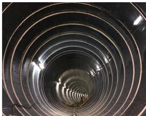
Fig. 1. Photograph of a steel plate reinforced segmental tunnel lining.
