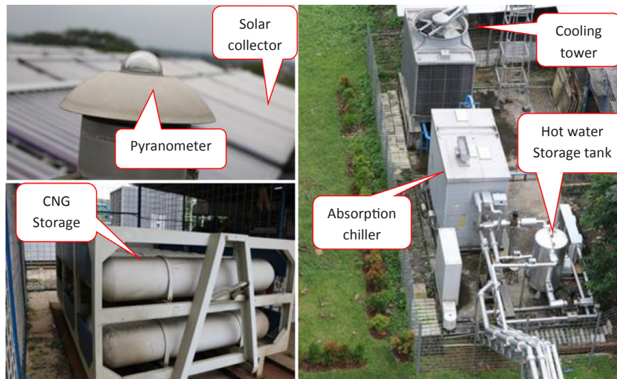
Fig. 1. Absorption chiller components.
