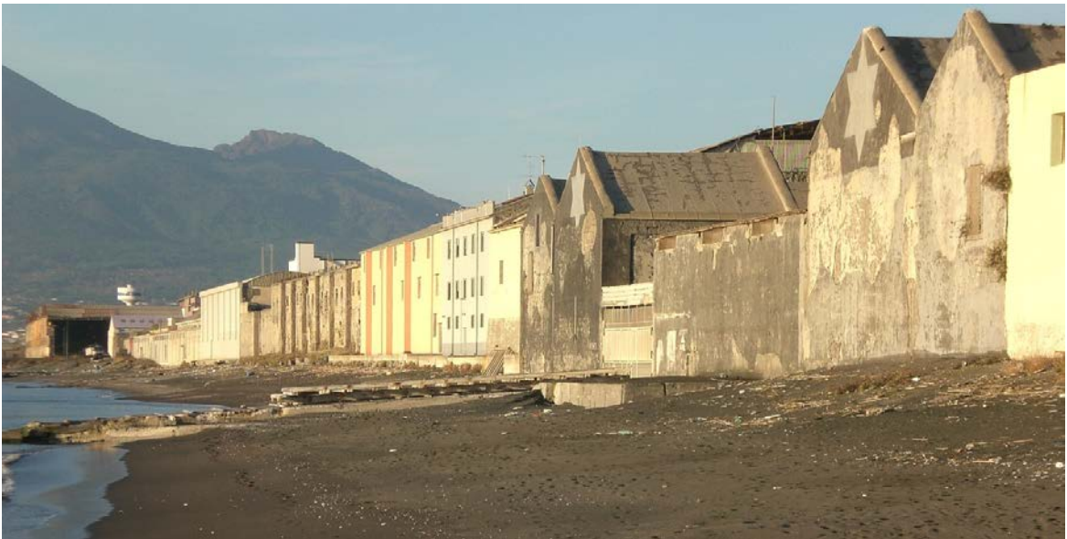
Fig. 1. Waterfront of Castellammare di Stabia: industrial warehouses along via De Gasperi
