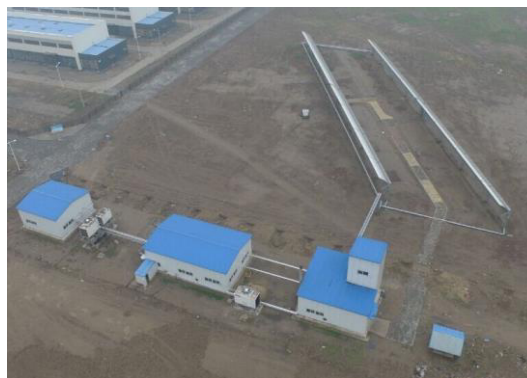
Fig. 1. Full view of the solar power plant
