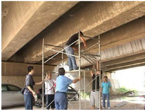
a) Inspection on the scaffolding
