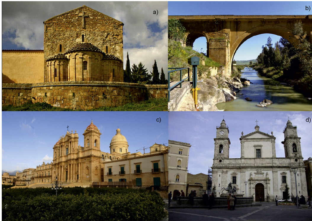
Fig. 1. The use of Sabucina Stone in some representative monuments of southern Italy. (a) S. Spirito church; Caltanissetta (1151); (b) Capodarso bridge (1556); (c) Noto Cathedral (1703–2007); (d) Caltanissetta Cathedral.
