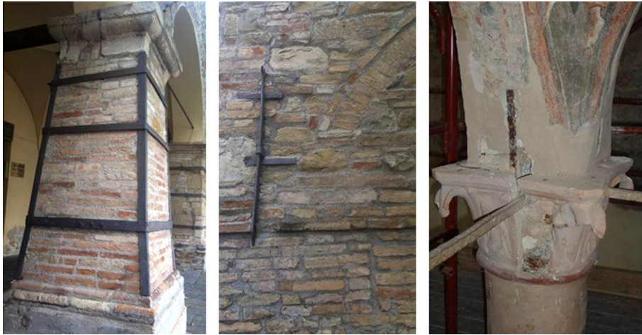
Fig. 1. Examples of use of metal inserts in cultural heritage buildings.
