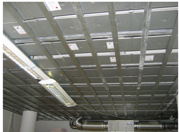
Fig. 2. Installation of the PCM boards in the conference room in Würzburg.
