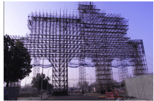
Fig. 2. Construction process of the Seville Fair Gateway, 2011.
