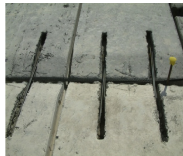
(b) Examples of horizontal ties
