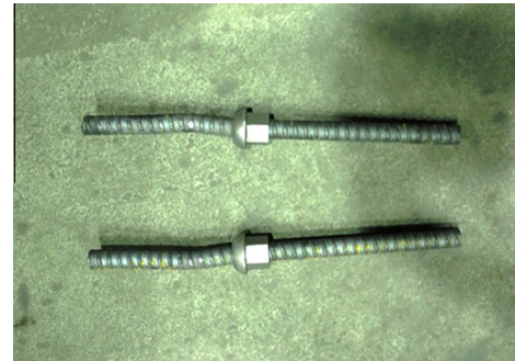
Fig. 4. Angled bolts showing shear damage caused by the tension in the cross member.
