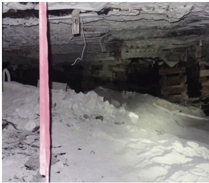
Fig. 2. Floor heave in the area without support.
