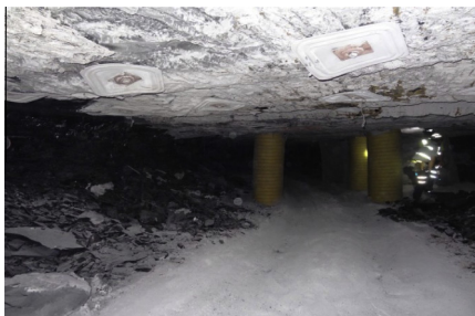
Fig. 3. Rib failure and spalling.
