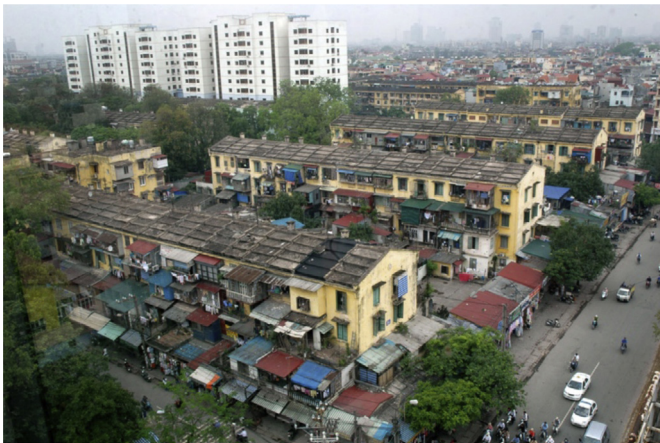
Fig. 1. Ha Noi worker housing built in the 1960's.
