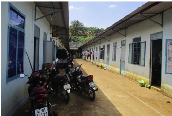
Fig. 2. One-story boarding house worker housing type.
