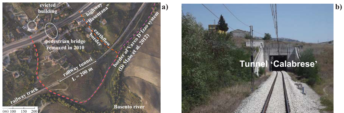
Fig. 1. a) Map with location of study area and railway tunnel, and with indication of main damages due to the landslide; b) Front view of railway tunnel “Calabrese”.
