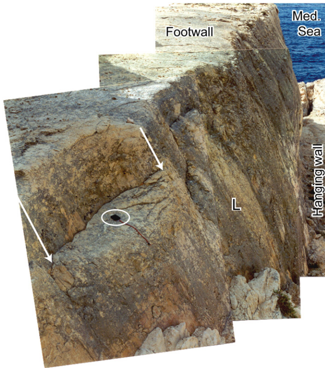
Fig. 1. Fault with a displacement of 11 m offsetting a limestone sequence at Il-Blata, SW Malta (Photo: C.G. Bonson). The fault surface dips steeply to the right and the upper surface of the limestone bed in the footwall and hanging wall are labelled. Arrows indicate the displacement of a lens within the fault zone and a lens of limestone breccia is also labelled (L). The cuspate shape of the footwall cut-off and irregularity of the fault surface is attributed to excision of limestone lenses, possibly the result of fault dip refraction (the much weaker Globigerina Limestone overlying the massive Lower Coralline limestone pictured here has been eroded).
