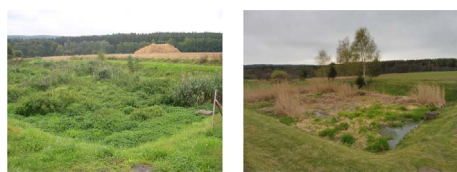
1993 Average outflow concentrations 2016 BOD 5 : 3.8 mg l -1 , COD: 22 mg l -1 , TSS: 3.2 mg l -1 BOD 5 : 4.0 mg l -1 , COD: 20 mg l -1 , TSS: 3.8 mg l -1
