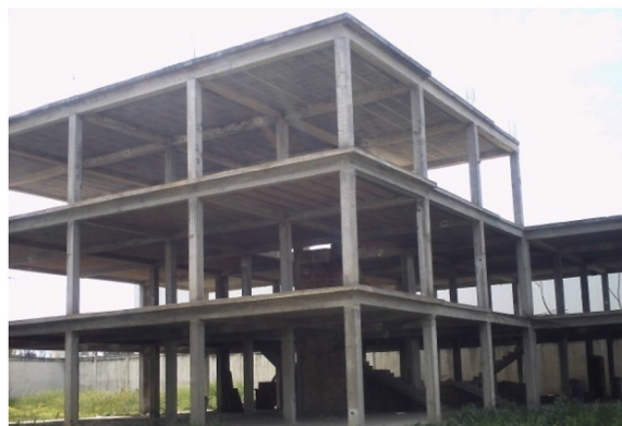
Fig. 1. Study case of an existing building.
