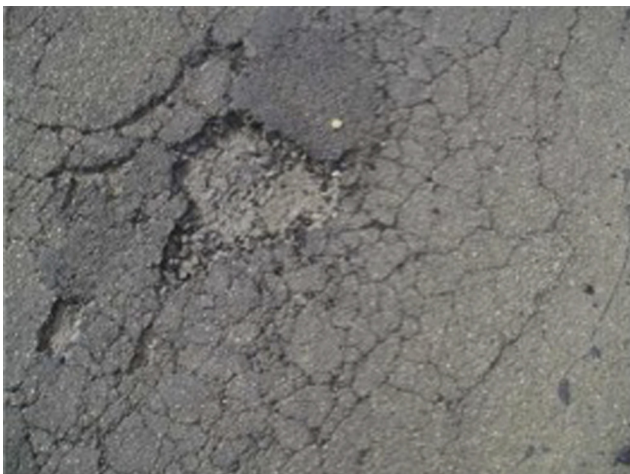
Fig. 1. Wear losses on pavements by aging effect.
