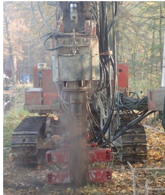
Fig. 2. Drilling equipment of traditional injection [authors].
