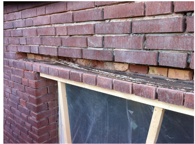
Fig. 2. Retrofitting of window beam with corroding bed joint reinforcement.
