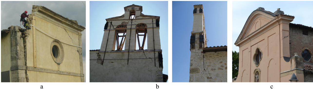
Fig. 1. Occurred damage to standing structures after L'Aquila earthquake, 2009 (a, b) and the Emilian earthquake, 2012 (c): (a) Santa Maria degli Angeli church (Civita di Bagno, AQ); (b) San Michele Arcangelo church (Villa Sant'Angelo, AQ); (c) San Francesco d'Assisi Church (Finale Emilia, MO).
