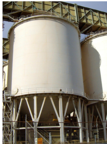
b. 10,000 ton steel grain storage, Australia [2]
