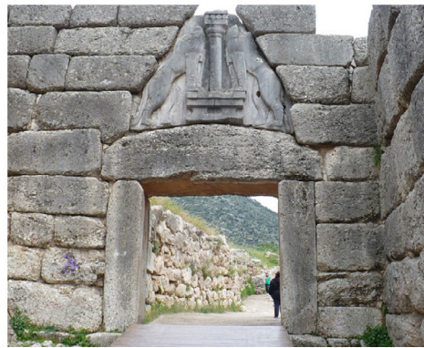
(c) Ancient Greek stone masonry construction with dry joints in Mykenes, Greece
