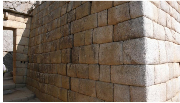
(b) Classical Inca architectural style of polished dry-stone walls of regular shape in Machu Piccu, Peru
