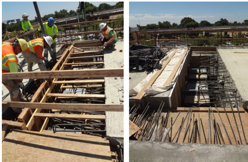
Fig. 2. Construction of in-span hinges in CIP/PS box girder bridge.
