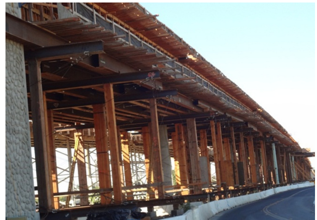
Fig. 4. Bridge falsework (Del Paso Park Overhead, Sacramento).
