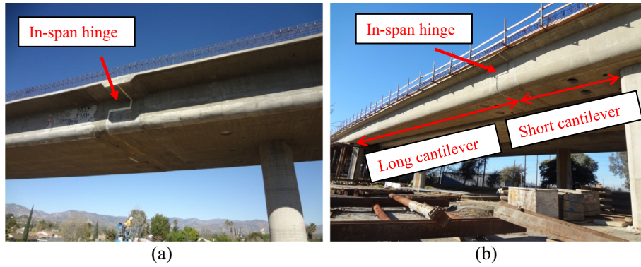
Fig. 1. (a) In-span hinge of CIP/PS box girder bridges (N170-N5 Connector, Los Angeles); (b) hinge span (Del Paso Park Overhead, Sacramento).
