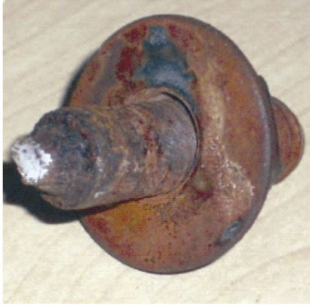
Fig. 1. Corroded and failed roof bolt.
