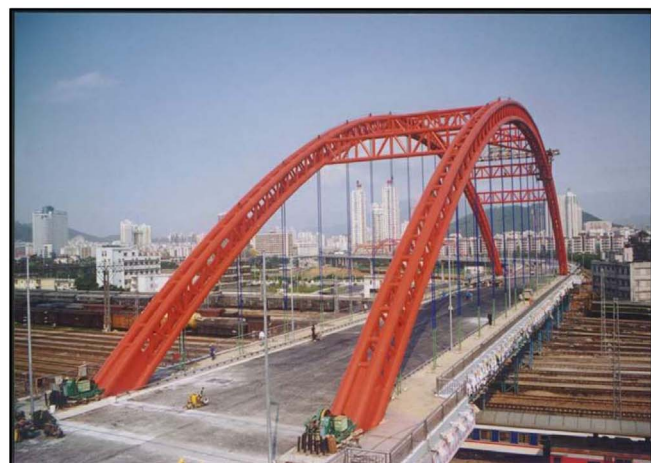
(c) Truss CCFST type
