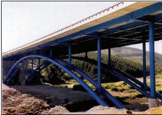
(a) Single-tube CCFST type
