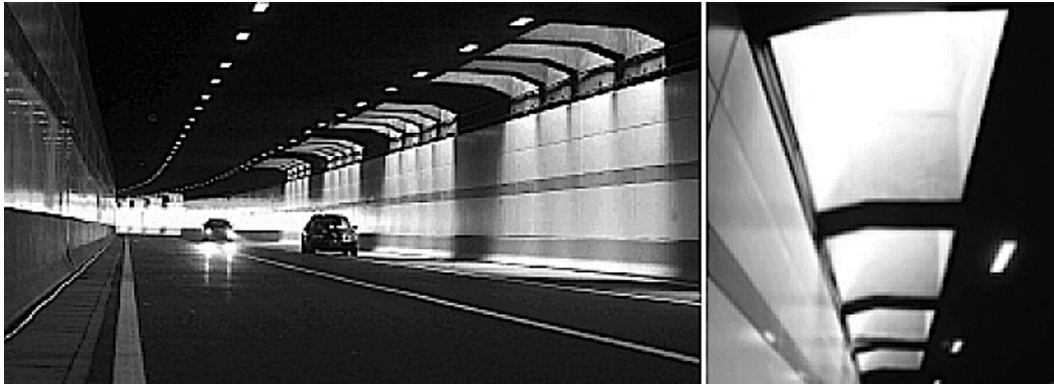
Fig. 1. Nanjing Xi'anmen Tunnel with roof opening.
