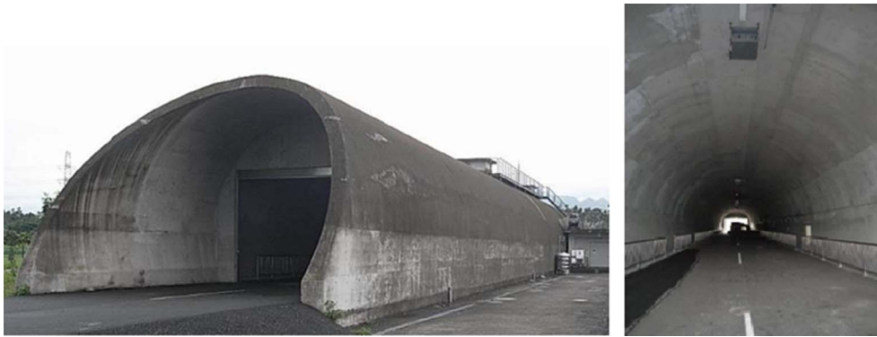
Fig. 1. NFA tunnel is 80 m long, 10 m wide and 6.5 m high.
