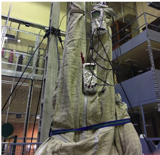
Fig. 2. Dangerous and inaccurate way of leakage current measurement by “shielded” micro-ammeters.
