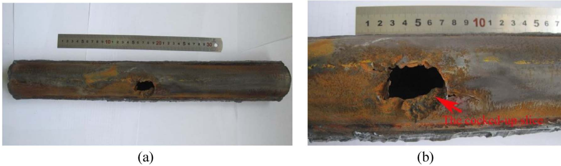
Fig 1. General view of the failed tube (a) and the enlarged view of the fracture (b).
