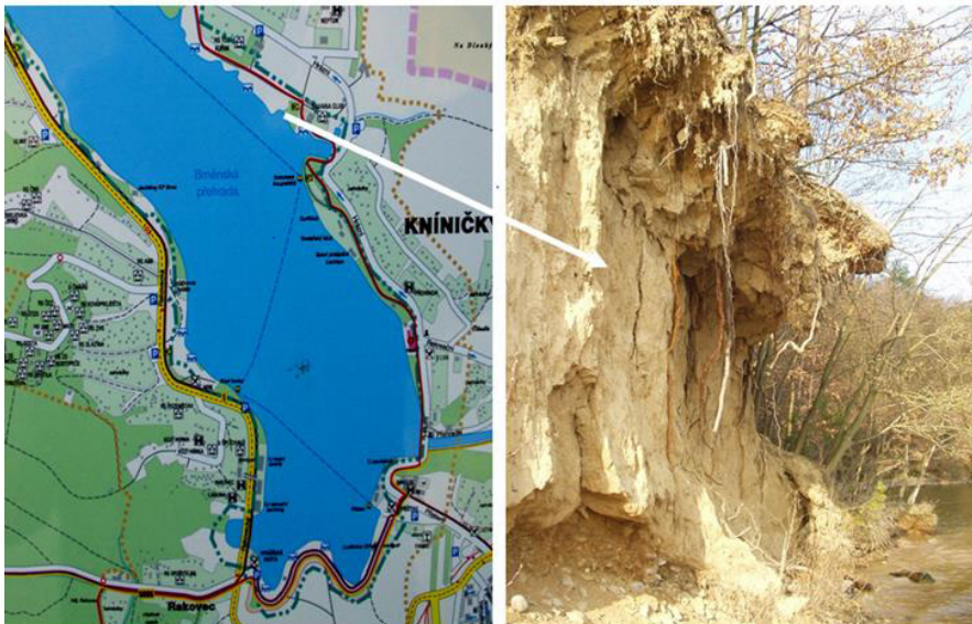
Fig. 1.(a). Brno Reservoir – (b) bank damage.
