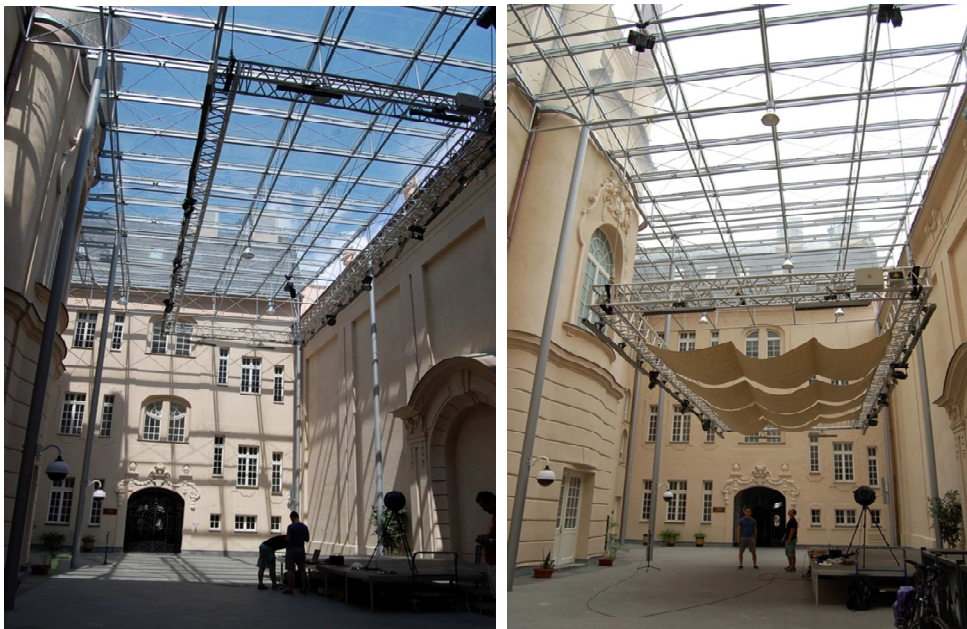
Fig. 1. Interior of the atrium of Slovak philharmonic in Bratislava with and without absorptive material placed over the stage
