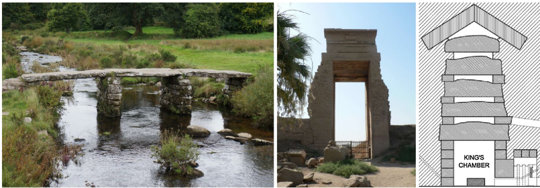
Fig. 1. Examples of stone beams from left to right: the clapper bridge at Postbridge (XIII century, span 3.75 m); the Nectanebos II gate at Karnak (the unsupported length of the beams is 7.2 m; note the relieving gaps between the beams); the relieving chambers inside the great pyramid of Cheops, where granite beams span 5.2 m.
