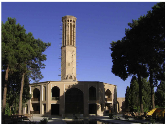
Fig. 1. The wind catcher of Dolat Abad Garden in Yazd (a central city of Iran).
