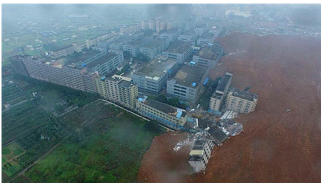
Fig. 3. Destroyed buildings engulfed by the Shenzhen landslide, Image is from www.baidu.com .
