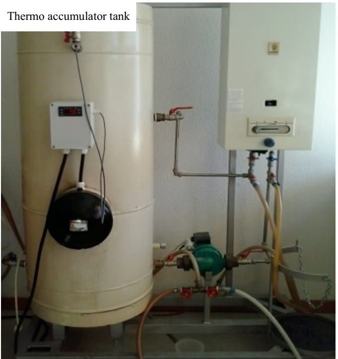
Fig. 2. Heating water system.
