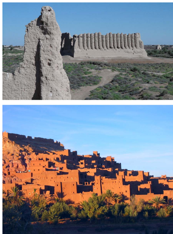
Fig. 1. Two notable old earthen structures: (upper photo) The ruins of Persian rammed-earth fortress, the Greater Kyz Kala, built in the sixth century CE for defense purpose in Merv, Turkmenistan. Photo attribution: Creative Commons, by Hergit, CC BY-SA 3.0, created 16 September 2011. https://en.wikipedia.org/wiki/Merv . (lower photo) The Ksar of Ait-Ben-Haddou in Ouarzazate province in south Morocco is a sprawling earthen structure built for fortification in the seventeenth century. Photo attribution: Creative Commons, by Donar Reiskoffer, CC BY-SA 3.0, created 14 December 2005, https://en.wikipedia.org/wiki/A%C3%Aft_Benhaddou .
