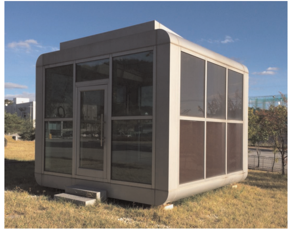
Fig. 1. Solar cube installed by the fabricated a-Si:H semi-transparent GTG PV modules.
