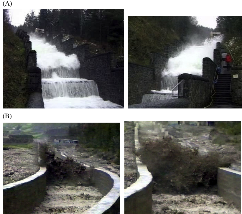
Fig. 1. Surge instabilities in high-velocity open channel flows (A) free-surface instability down the Sorpe dam spillway, Germany in 2003 (Courtesy of Ruhrverband) – \theta = 18^\circ , h = 0.5\text{--}2 m (pooled steps), Q = 6.9 m 3 /s, Re = 1 \times 10^6 and (B) air–water–sediment surges down a channelised section of Rio Achumani, La Paz, Bolivia in 1993 (Courtesy of Francis Fruchard) – Flat step design.
