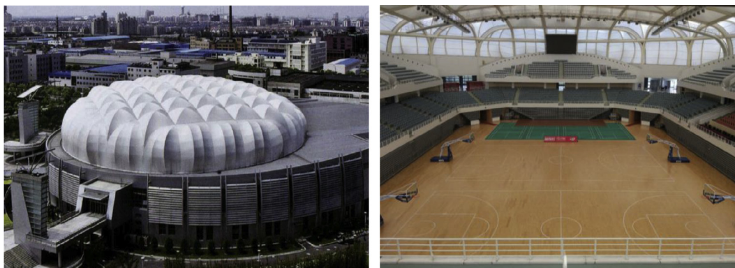
Fig. 1. Bird's eye view and indoor pictures of the enclosed large-span membrane building.
