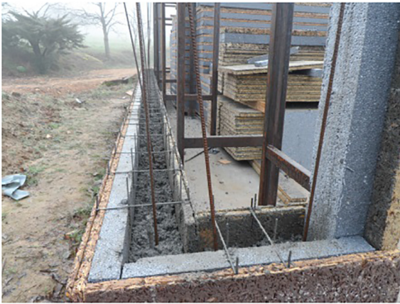
Fig. 1. Wood cement panels as permanent formwork.
