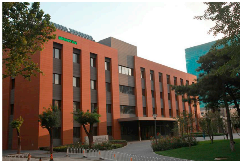
Fig. 1. North Façade of CABR Nearly Zero Energy Building.
