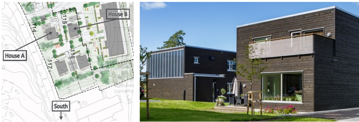
Fig. 1. Left: site map of Rudshagen passive houses. Right: the two passive houses that are measured in the present study: House B with the heat pump at the r.h.s. and the solar heated House A at the l.h.s. (photo: Tove Lauluten).
