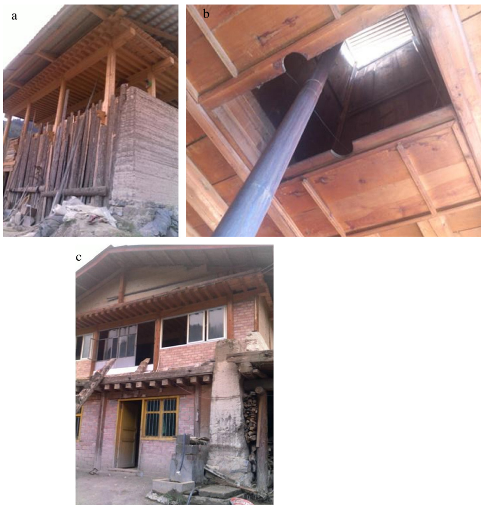
Fig. 1. Tibetan traditional dwellings: (a) two-story wooden framework; (b) flue channel; (c) outside view.
