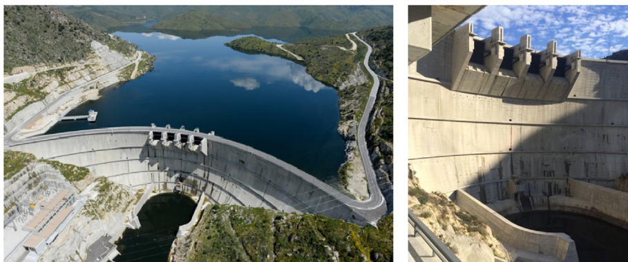
Fig. 1. Baixo Sabor arch dam, aerial view of dam and reservoir and detail of the spillway from downstream [22].
