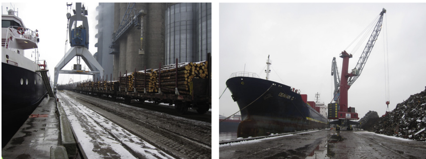
Fig. 1. Examples of vertical loads on quay decks.
