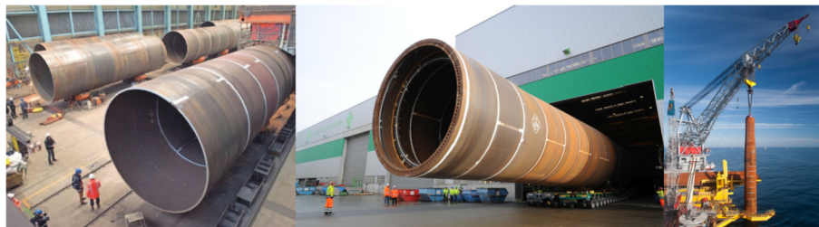
Fig. 1. Fabrication and on-site setting up of monopile type support structures for an offshore wind farm (source: Heavylift news, OffshoreWIND.biz, Groundsure Location Intelligence).
