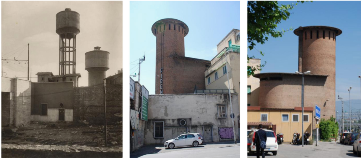
Fig. 1. Photographic view of the two tanks before the construction of the encasing masonry building (in 1935) and current views of the latter from the same and the opposite viewpoint.
